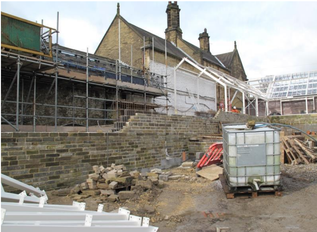
Work in progress, March 2017; photograph by David Quail
